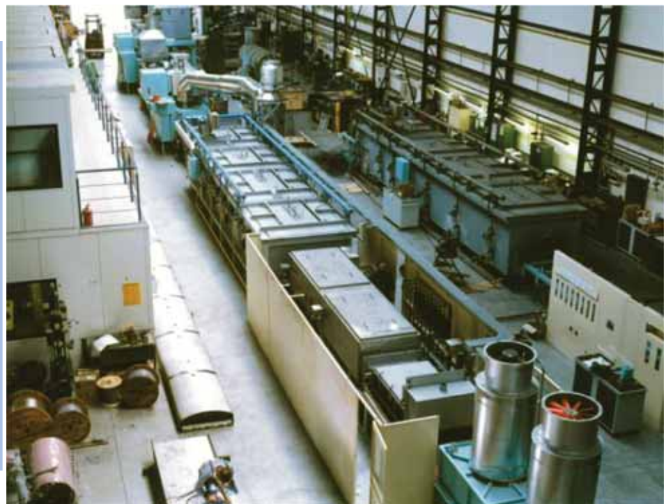
Overhead view of CAB furnace line under construction
