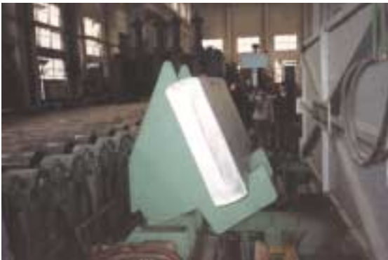
Discharge end with ingot down-ender and mill roll table
