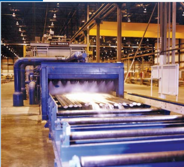
Solution Heat Treat Furnace with spray quenching for aluminum extrusions
