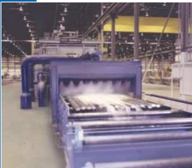
Solution Heat Treat Furnace with Spray Quenching for aluminum extrusions
