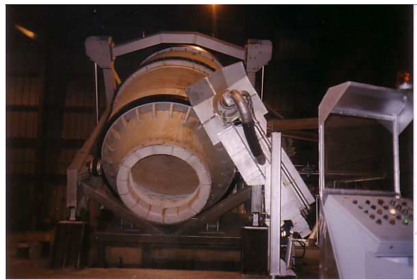
Photo 7: Burner Door Assembly
