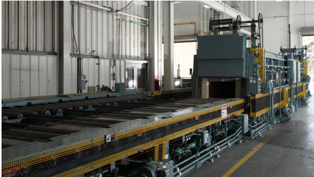
Figure 3 - Roller Hearth furnace system for heating, reheating and air annealing
