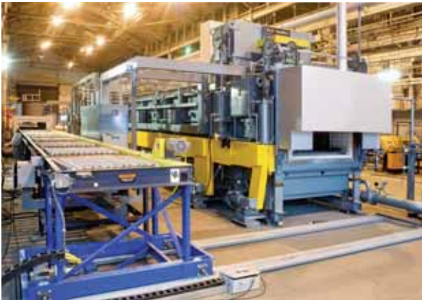
Roller Hearth – Transformer Core Annealing
