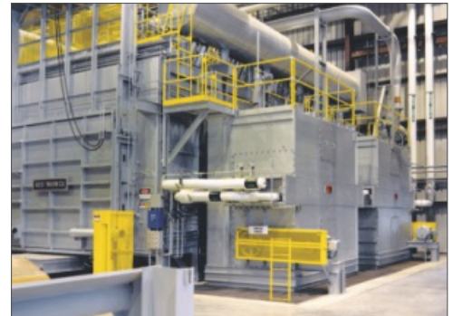
Bypass cooler reduces fin maintenance and keeps performance at peak levels
