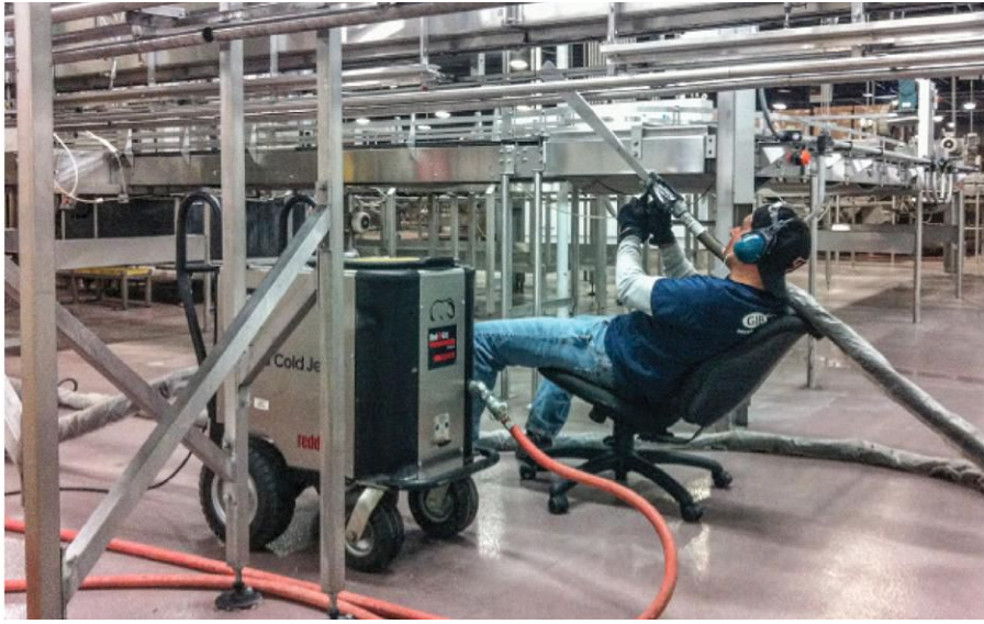
Fig. 1. Ice blasting of heat-recovery steam-generator components
